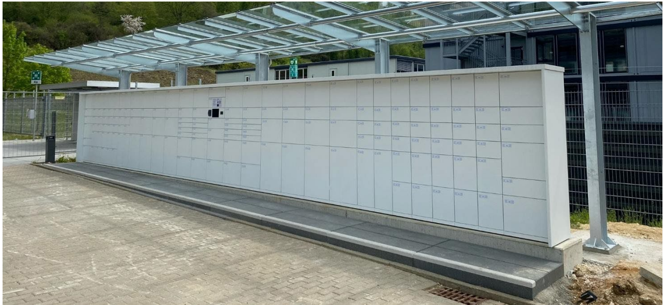
Fig. 114 Example of an outdoor parcel box system
